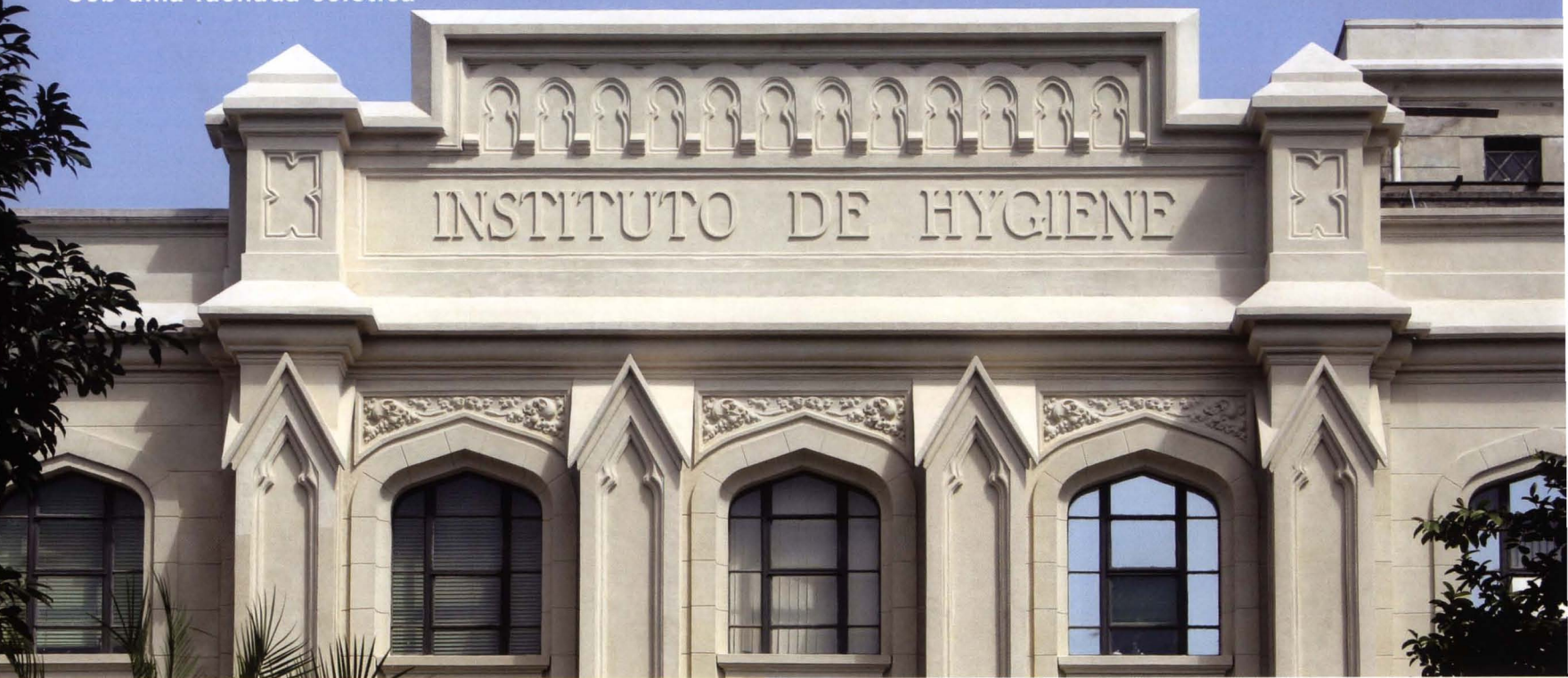
Fachada restaurada: elementos preservados The restored facade: details were preserved
