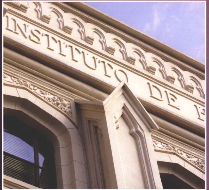
Fachada do primeiro prédio durante as obras e depois de pronta The facade of the first building during the work and after completion.
